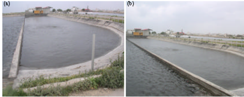
Fig. 2: Two views of the existing settling channel and polishing pond
