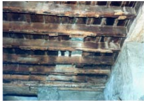
Fig. 1: Repair of old stringers with traditional methods
