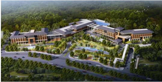
Fig. 3: The design picture of the entrance area at the site of Tennis-badminton Center Club (Source: designed by writers)
