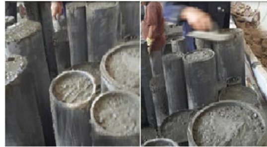
Fig. 4: Casting the composite columns
