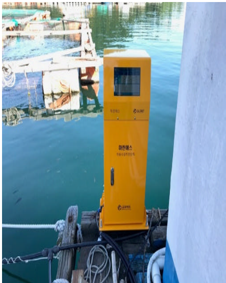
Fig. 3: Marine-S smart water quality measuring sense
