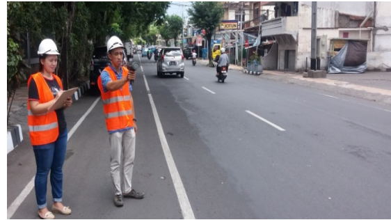
Fig. 3: Documentation of Sam Ratulangi Street in Manado city (Sta 2+000-2+200 segment)
