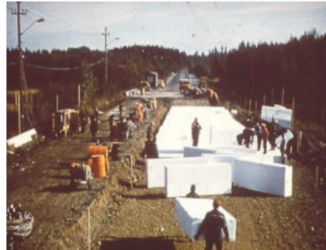
Fig. 1: Road construction using EPS block
