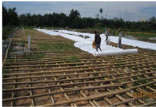
Fig. 5: Ground improvement using bamboo grid frame technology
