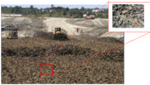
Fig. 2: Tire shreds into 50-300 mm in length
