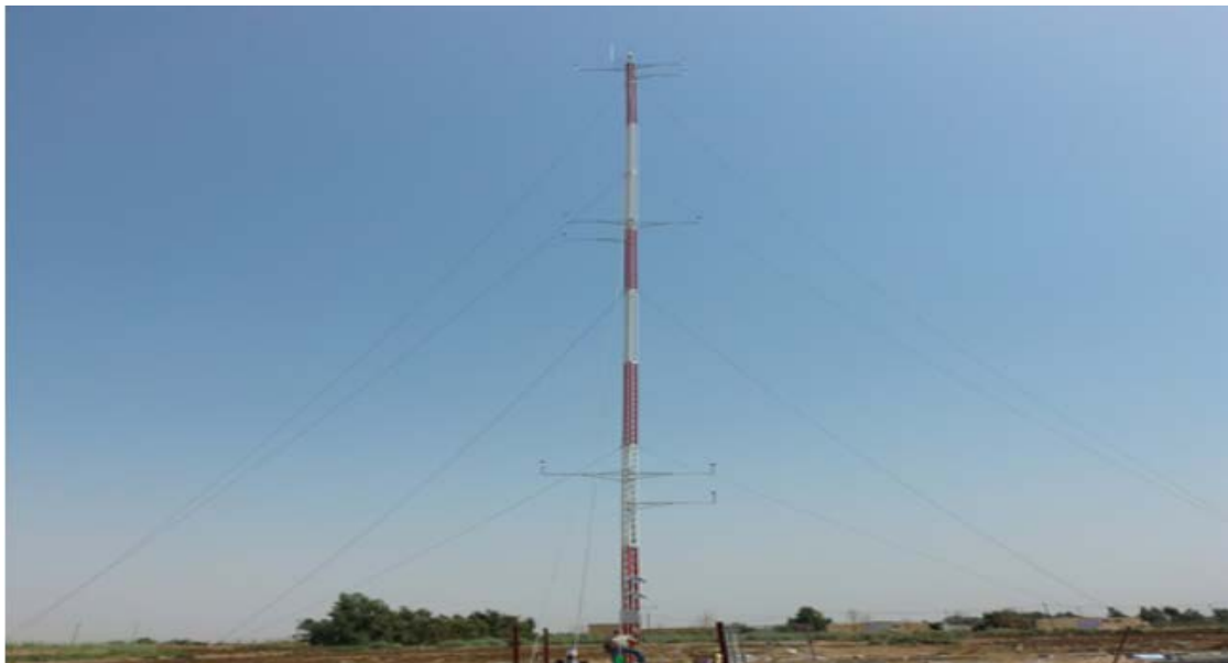
Fig. 4: The aerial tower
