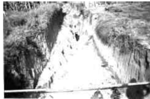
Fig. 3: An abandoned chmelisation project overtaken by gullies in a downslope position currently undergoing various developments (site B in Fig. 1). An exposed pipe and the author were shown at the background
