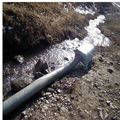
Fig. 4: Appearance of derivative micro HPP with pressure hose
