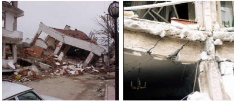
Fig. 1: Examples of cases -Severely damaged-SD
