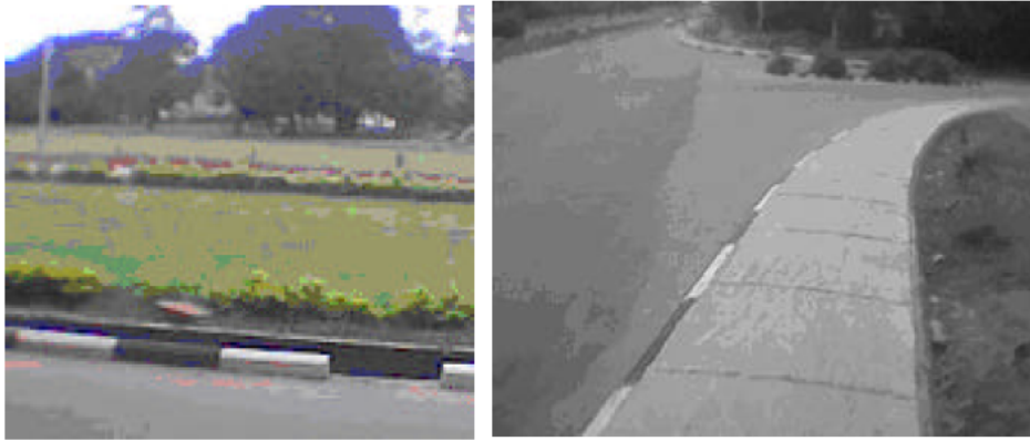
Fig. 2: Well maintained roads
