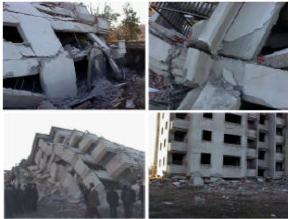
Fig. 8: Damaged multistory structure
