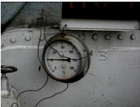
Fig. 10: A temperature gauge attached to MC1/S125 blending tank
