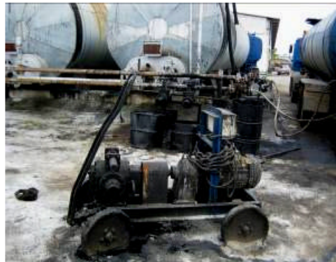
Fig. 9: Special pump used to circulate cutback asphalt mixture
