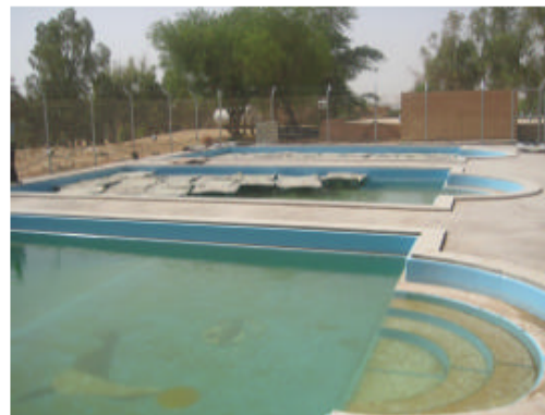
Fig. 2: General view of pools and the site used for the study
