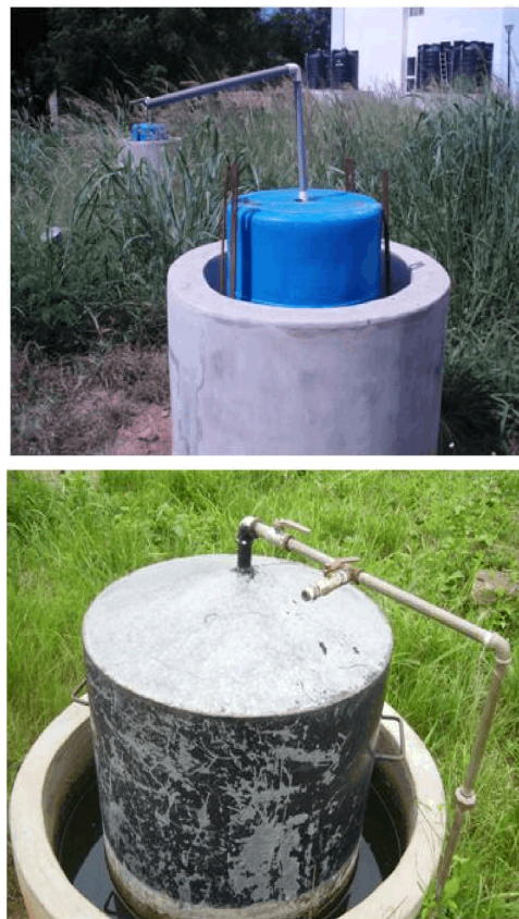
Fig. 6: (a) A Broken down twin floating-drum plant at GIMPA; (b) Abandoned floating-drum plant at Tepa slaughterhouse
