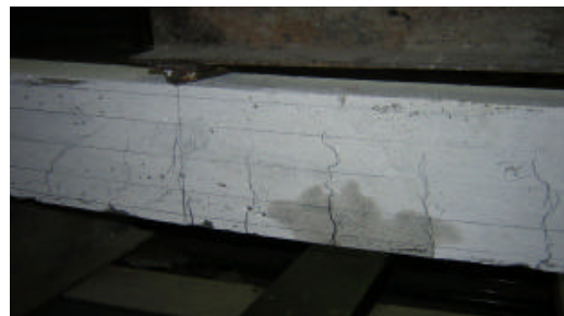
Fig. 5: Failure pattern of the GFRP beam
