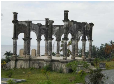
Fig. 2: Existing condition of the Bale Kapal
