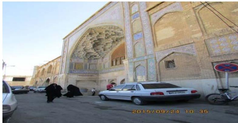
Fig. 3: The exterior of the school Khan, Shiraz (Riahi, 2015)
