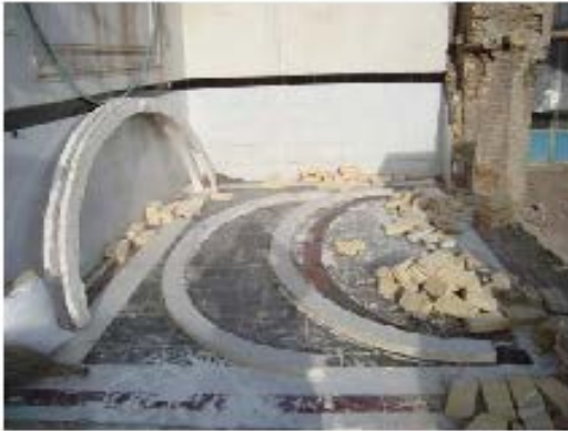
Fig. 12: Implementation of groin with plaster stencil (Aniran in 1392)
