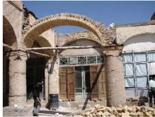
Fig. 19: Using Cache beam in groins of Saraye Dokhan of Zanjan (Aniran in 1392)
