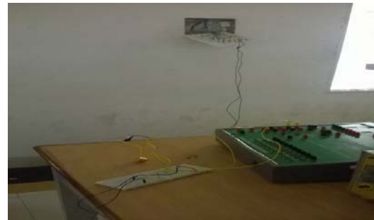
Fig. 15: A relay circuit connected to FPGA to control Appliances
