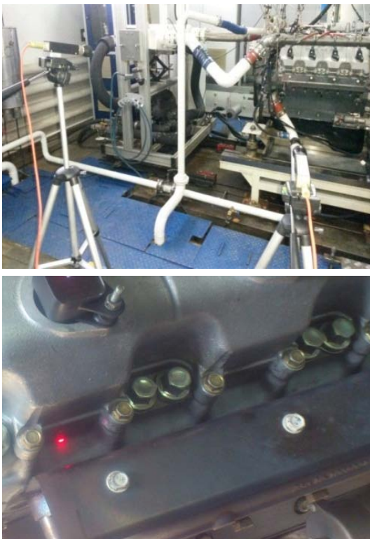
Fig. 14: Installation of laser vibrometers (left) and place the guidance of the laser vibrometer at the head of the gas engine block (right)
