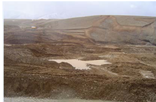
Fig. 4: View of the under construction dam site conglomerate of Eyvashan
