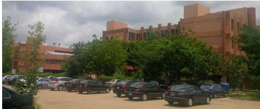
Fig. 3: Federal secretariat complex, bauchi, Nigeria (Adeyami et al. , 2015)
