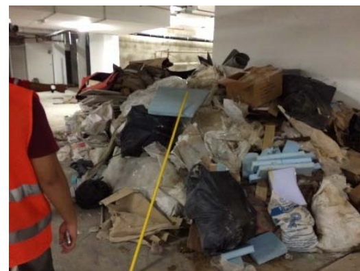
Fig. 2: Inadequate risk assessment
