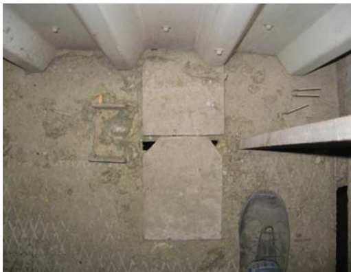
Fig. 6: The gap between the stops, the ends of the stops are not planed
