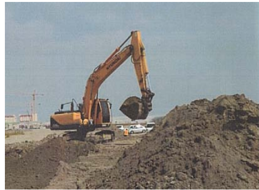
Fig. 3:Construction of road with consolation soil
