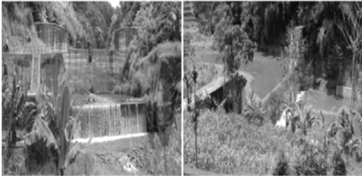
Fig. 4: Examples of check dams in the upper reach of the Brantas River
