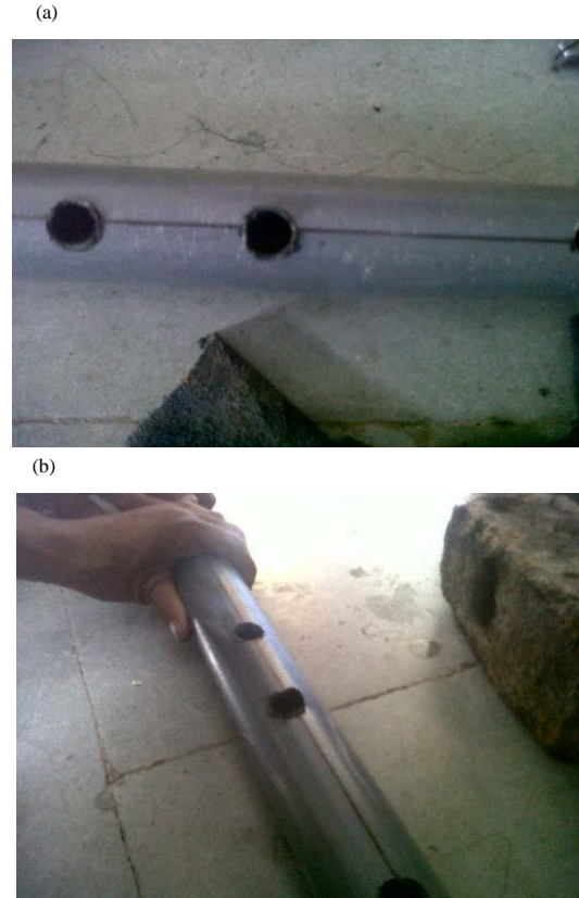
Fig. 4: a, b) Header pipe marking and drilling holes for other pipes
