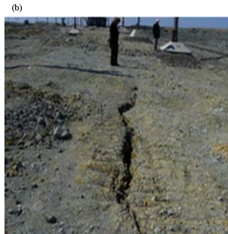
Fig. 3: a) The deformations on the ground surface and b) The engineering structures
