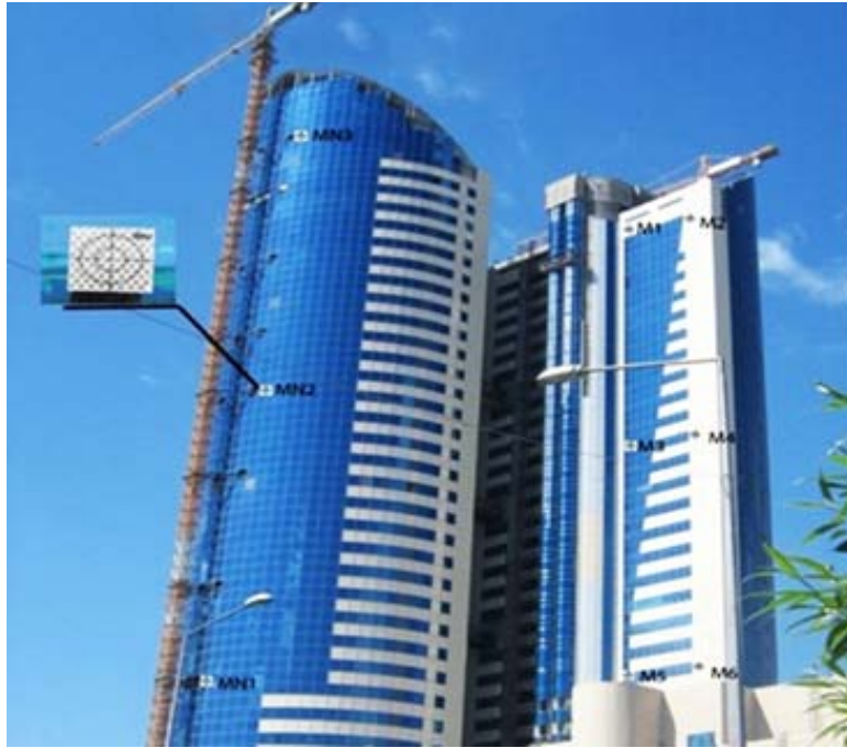
Fig. 5: Location of the benchmarks on the object “KTZ Administrative building”
