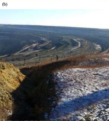
Fig. 2: a) The Southwestern side of the open-cast and b) Cracks with wide opening up to 1.5 m
