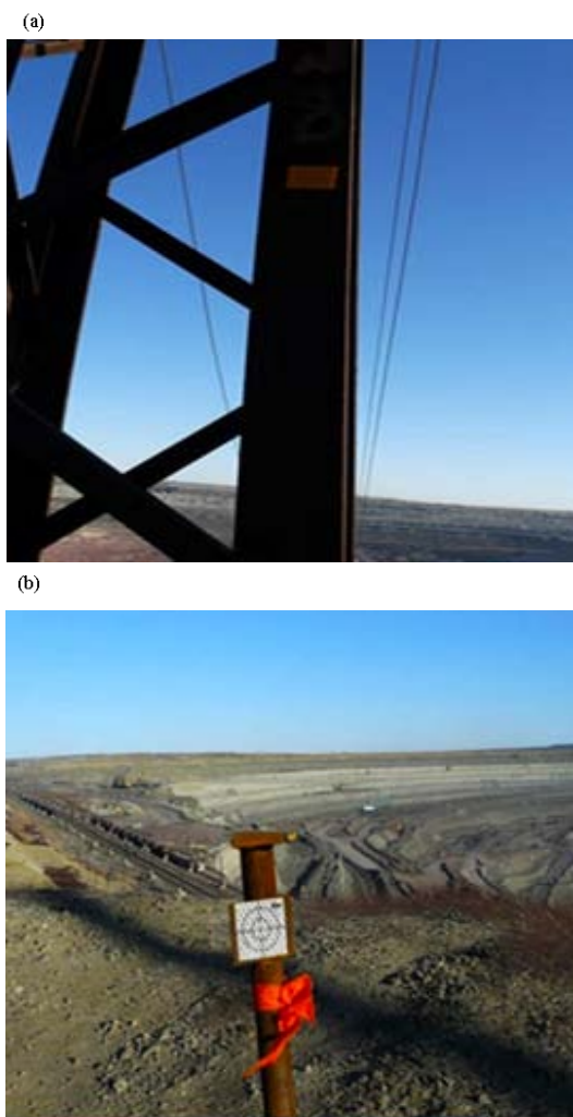
Fig. 8: a) The deformation control benchmarks were installed in September, 2011 on the ETL supports and b) Caving coil in the monitoring station No. 1 area
