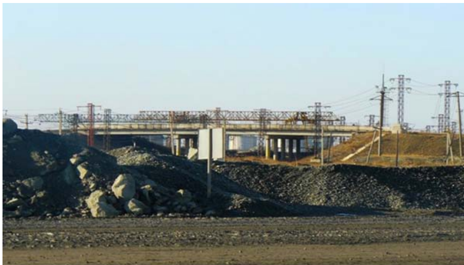
Fig. 4: The overpass of the industrial site of the open-cast in the Maykain mining affected area
