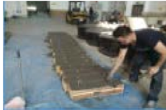
Fig. 1: Concrete casting of RC beam
