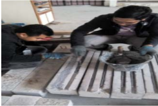
Fig. 3: Beam specimens with complete grooves ready for GFRP installation
