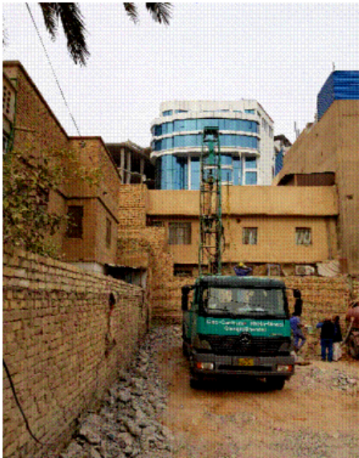
Fig. 2: The drilling machine which was used in boreholes drilling
