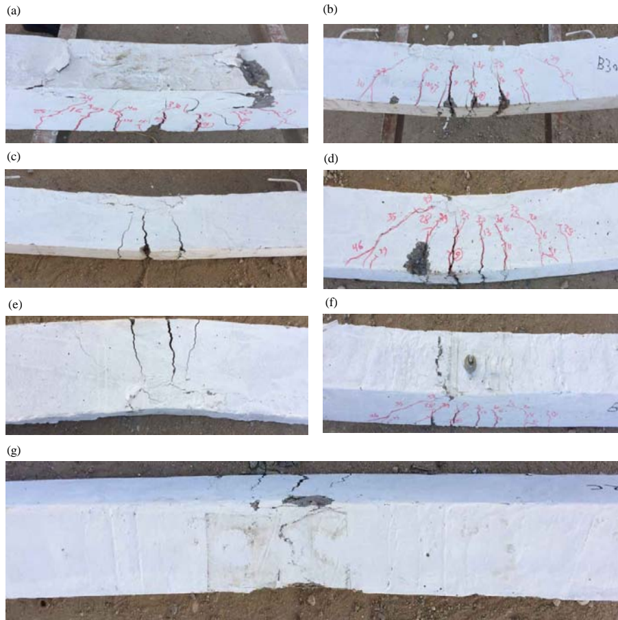
Fig. 14: Beams after failure: a) R30; b) B30; c) R20; d) B20; e) R10; f) B10 and g R
