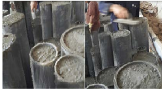
Fig. 4: Casting the composite columns
