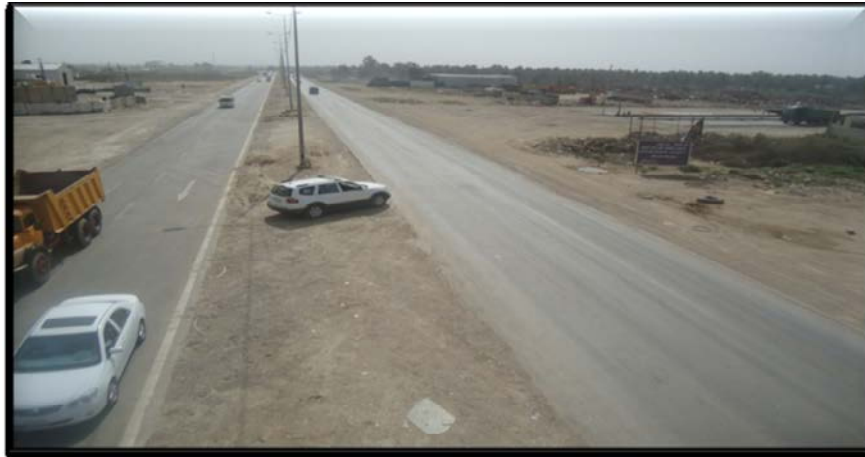
Fig. 1: The section of the roadway with illegally turning movement in the study area
