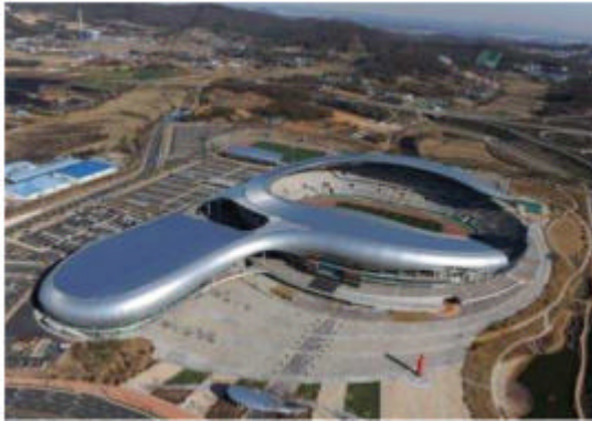
Fig. 1: Hwasung sports complex
