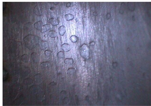
Fig. 3: Iron sulfide and underdeposit corrosion
