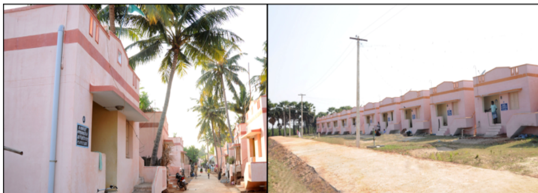
Fig. 7: Tsunami resettlement houses in Cuddalore
