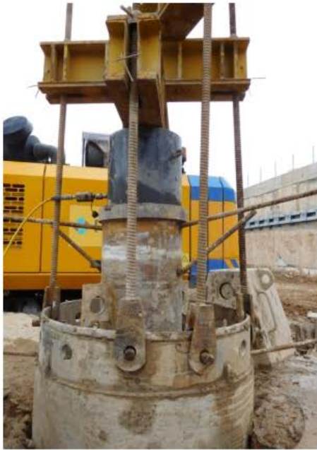
Fig. 19: Testing of piles on the principle of “pipe in a pipe”
