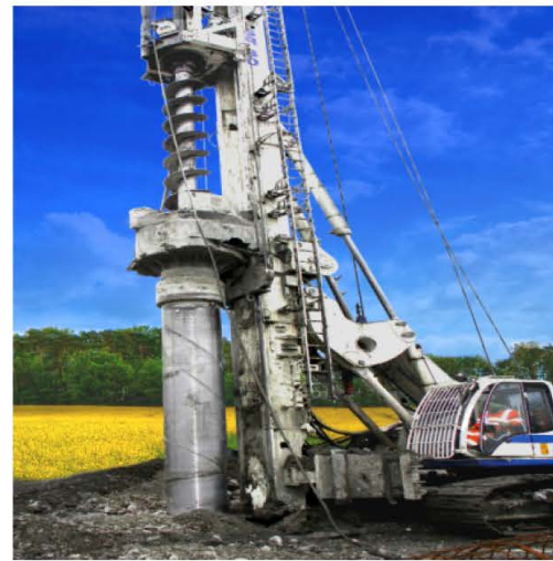
Fig. 15: Drilling rig for execution of the pile system CSP
