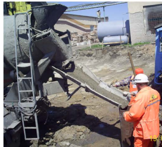
Fig. 10: Concreting of the casing shaft by mixer
