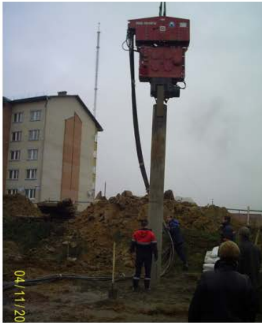
Fig. 11: Driving tapered casing by using hanging vibrohammer
