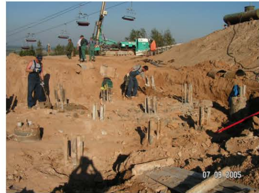
Fig. 17: Piles for end support cableway liftsnowboard in silich by inject technology (in the background can be seen the machine company (asagrande) to perform pile)
