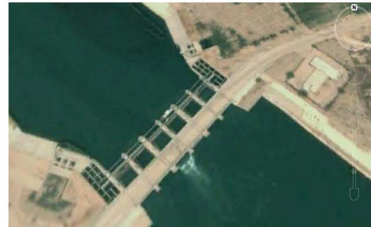
Fig. 2: The flood control structure under study
