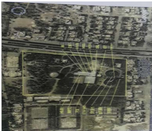
Fig. 1: Al-Tayyara water treatment plant
