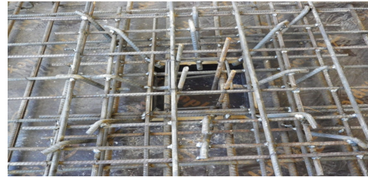
Fig. 4: Steel reinforcement mesh with perimeter swimmer bars
