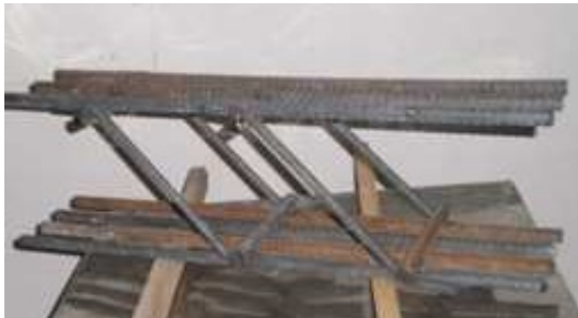
Fig. 2: Typical welded swimmer bars used in beams
