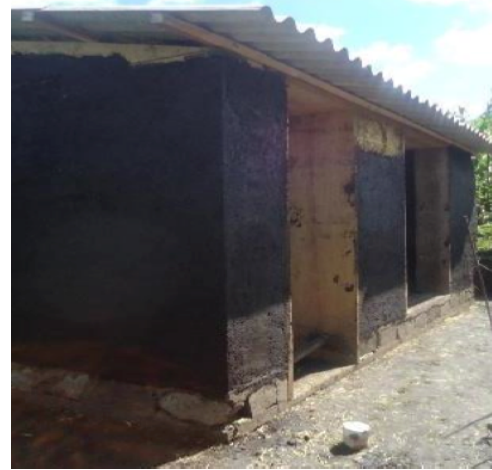
Fig. 14: Home with the plaster applied
