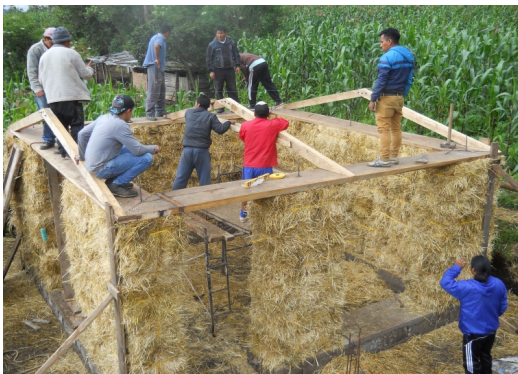
Fig. 13: Perimeter beams and wooden trusses
