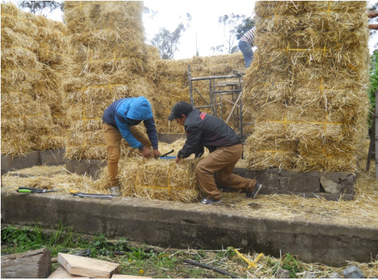
Fig. 11: Foundation and shaping of the structure's straw walls
