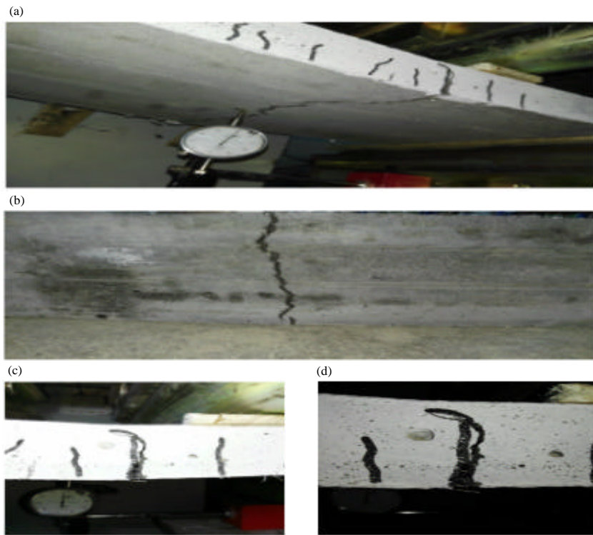
Fig. 18: a-d) Typical Failure of ferro geopolymer slab with steel fibers
