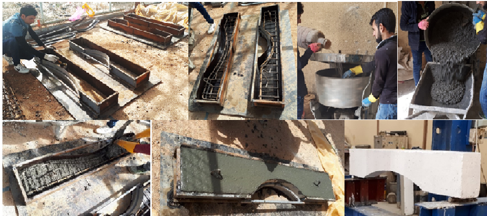
Fig. 4: Casting and curing process
