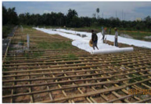
Fig. 5: Ground improvement using bamboo grid frame technology
