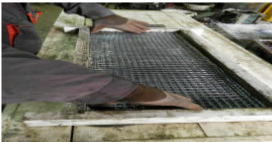
Fig. 4: Wire mesh installation in ferrocement layer
