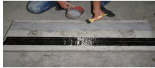
Fig. 5: Placement of CFRP sheets
