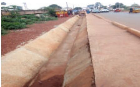
Fig. 16: Farm land along Odenigwe Road that dissipates fine particles into the drainage system during rain
