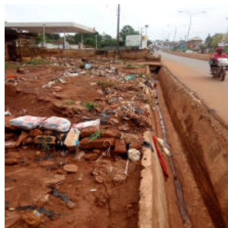
Fig. 20: Road with no temporary waste site, poor waste managements and poor drainage, e.g., University-Road
