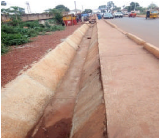
Fig. 6: Well-constructed drainage system in Enugu Road
