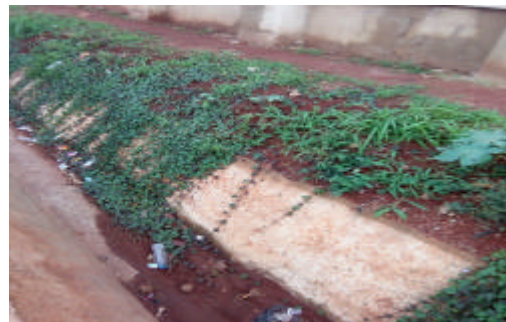
Fig. 14: Drainage section where latitudinal siltation should be prevented in Enugu-Road
