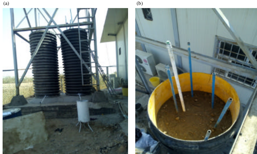
Fig. 1: a, b) Pilot scale lysimeters construction and filling
