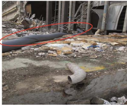
Fig. 8: Tube used for ammonia gas discharge
